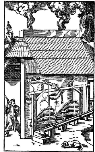
Figure 14: Backside of the smeltery with shaft furnaces, showing the bellows.
