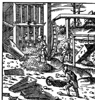
Figure 5: Screening of crushed ore.
